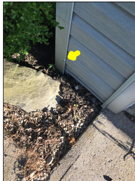
Holes along the siding.
