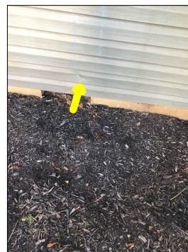
Damaged siding.
