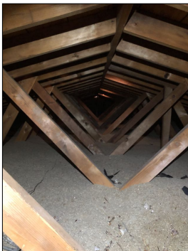
General photo of the attic.
