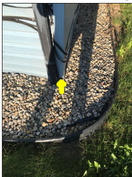
Damaged siding.
