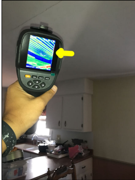
Operable heating elements.
