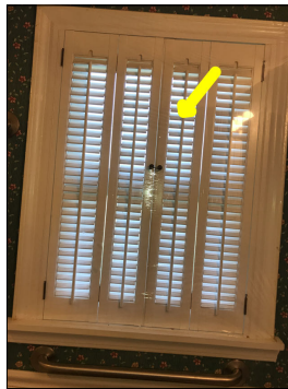
Unconventional plastic along the window. This is considered abnormal and a defect.
