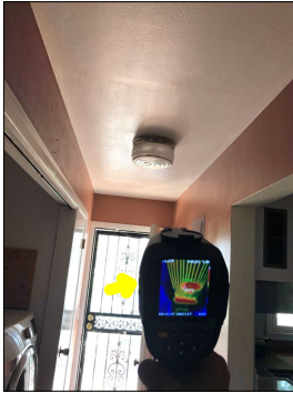
Operable heating elements.
