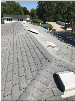
General photo of the roof.
