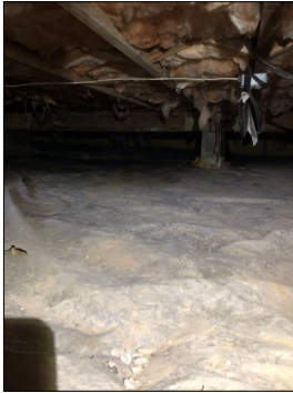
General photo of the crawl space.
