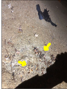
Signs of nesting/wildlife activity within the attic. Wildlife activity can cause property damage.
