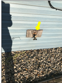
Holes along the siding.
