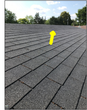
Unconventional waves/sags along the roof. This is considered abnormal and a defect.
