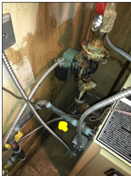
Discoloration along the wall. Discoloration along the wall is considered abnormal and a defect. An active or intermittent water source can cause discoloration, mold growth and property damage. Unconventional dirt/foreign substance along the wall behind the water heater. This appears to be wildlife/insect activity. This could also be structural with dirt coming in the wall. Recommend licensed contractor evaluate.
