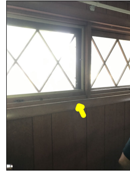
Broken/defective locks. Both locks have to be held open to open/close the windows. Aged windows. Window replacement should be anticipated.
