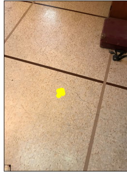
Crack along the foundation. Cracks are considered a defect. Cracks should be repaired/sealed to prevent the intrusion of moisture, insects, wood destroying insects, mice, and radon.
