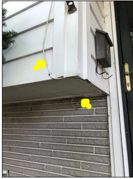
Loose wires along the house. These wires appear to be low voltage wires.
