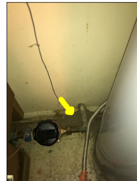
Discoloration along the wall. Discoloration along the wall is considered abnormal and a defect. An active or intermittent water source can cause discoloration, mold growth and property damage. Unconventional dirt/foreign substance along the wall behind the water heater. This appears to be wildlife/insect activity. This could also be structural with dirt coming in the wall. Recommend licensed contractor evaluate.
