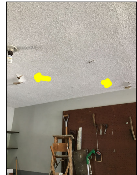
Flaking and peeling along the ceiling.
