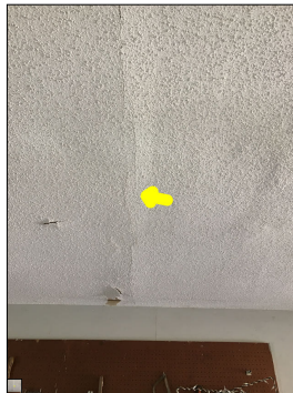
Cracks along the ceiling.
