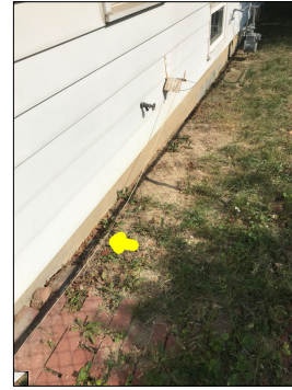
Loose wires along the house. These wires appear to be low voltage wires.
