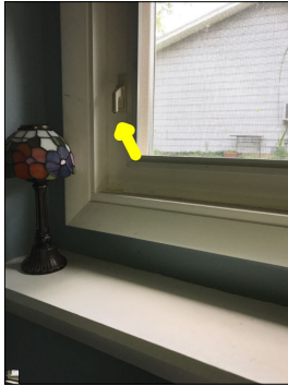
Broken/defective locks. Both locks have to be held open to open/close the windows. Aged windows. Window replacement should be anticipated.
