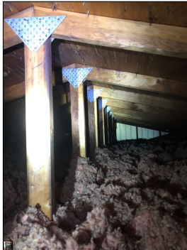
General photo of the attic.
