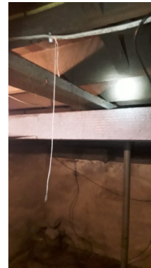
This is not the recommended install for a support. Missing anchors does not support on each end and easily shift left or right
