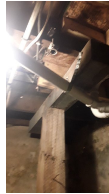
This is not the recommended install for a support. Missing anchors does not support on each end and easily shift left or right
