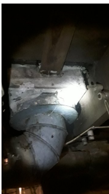
White tape, may contain asbestos.
