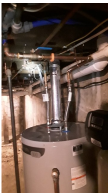
professional vent install.
