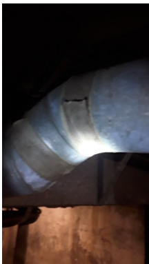
White tape, may contain asbestos.
