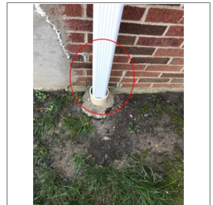
Cracks along the siding.
