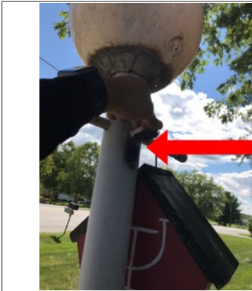
I was unable to get my receptacle tester in the receptacle. There is debris along the receptacle and debris within the receptacle. The debris is restricting the ability to plug something into the receptacle.
