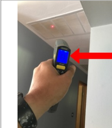
The photo identifies the temperature of the return air while the air conditioner was in operation. The approximate temperature of the return air was 67 degrees Fahrenheit.
