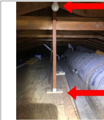
Apparent added support columns that go along the ridge line.
