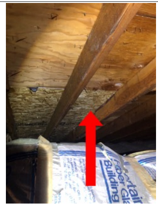
Several areas along the sheathing have been replaced.
