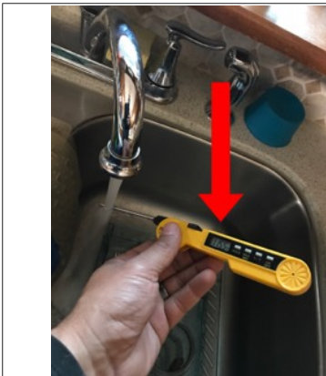
Temperature reading of the hot water during the time of the inspection. The approximate temperature of the hot water was 115 degrees Fahrenheit.
