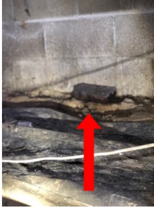
Pest control in the crawl space.
