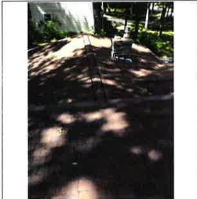
General photo of the roof.
