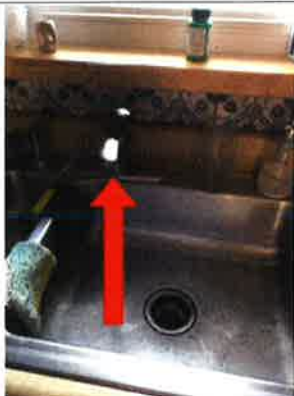
The faucet handle is difficult to move.
