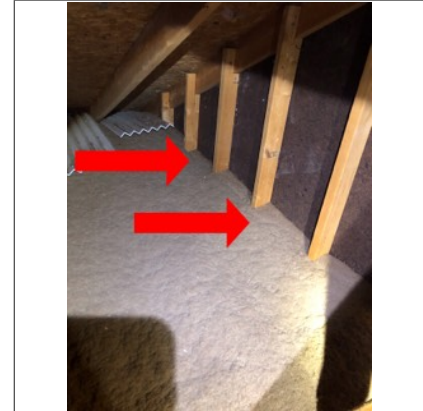
Mice/rodent tracks along the insulation.
