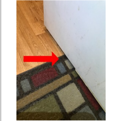
Torn weatherstrip along the entry door from the garage to the kitchen.
