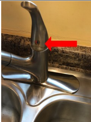
Corrosion along the faucet.
