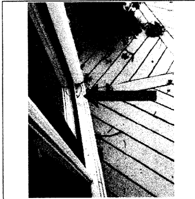
The screen door is missing.
