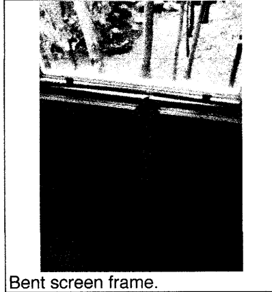
Bent screen frame.
