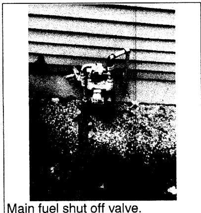
Main fuel shut off valve.
