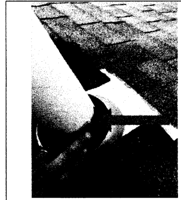
The flashing around the plumbing vent is torn. This is a potential leak point.
