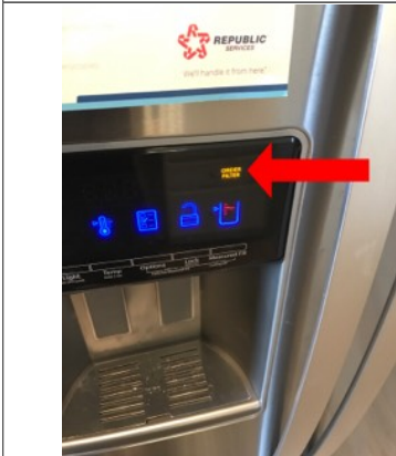
The filter needs to be replaced.
